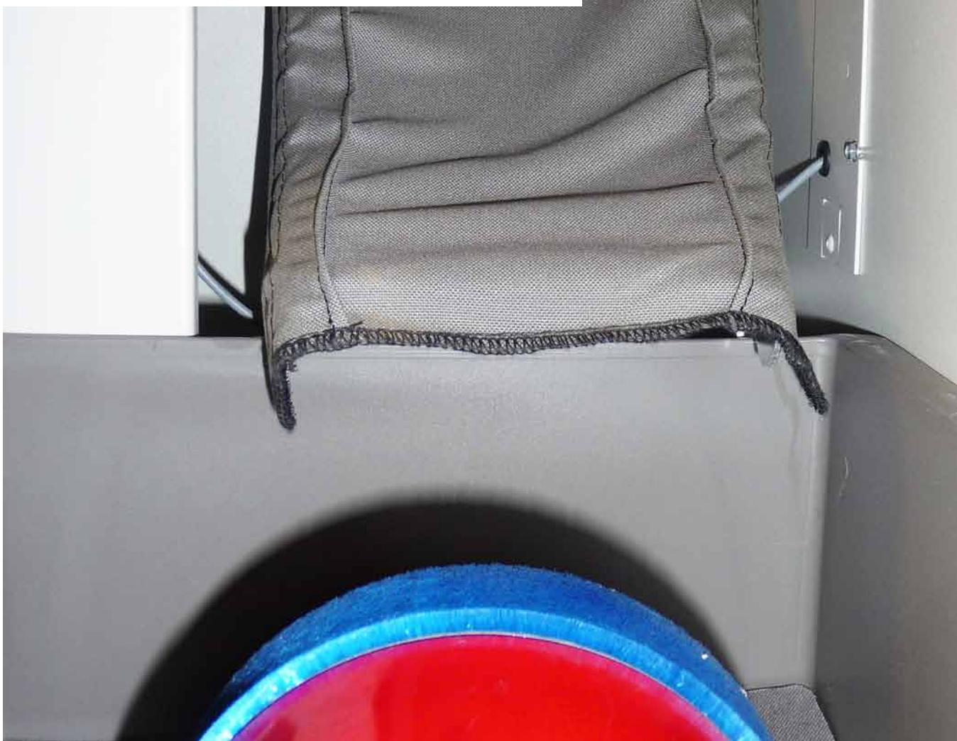
The Whisper Receiving System is available as an upgrade or as standard factory-installed equipment on new TransLogic 6-inch recessed PTS stations. Installation is quick and easy, and can be performed by hospital maintenance personnel or a Swisslog service technician for a fee.
